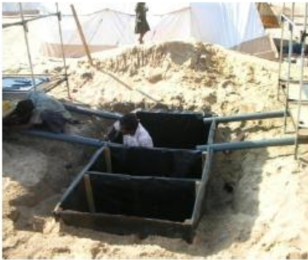
Assembling the prefab septic tank Photo UNICEF
